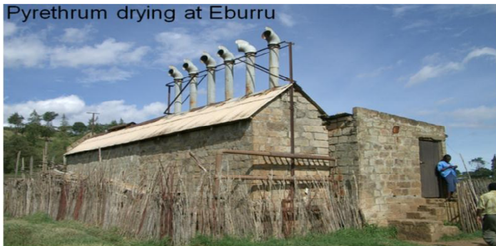
Figure 2.2: Geothermal energy being used by the local community at Eburru for pyrethrum drying.
