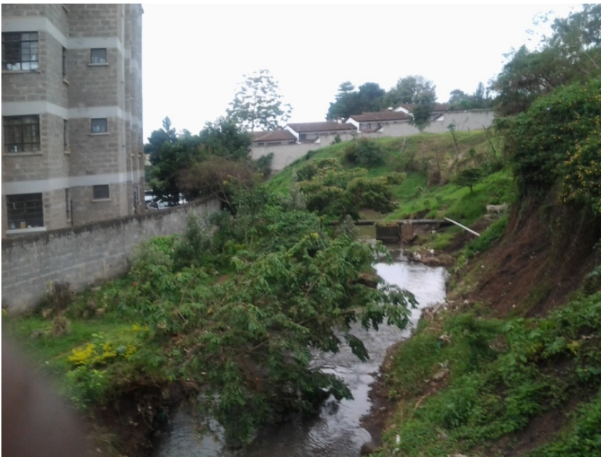
Plate 5.2 Encroachment on Kirichwa Kubwa riparian reserve
