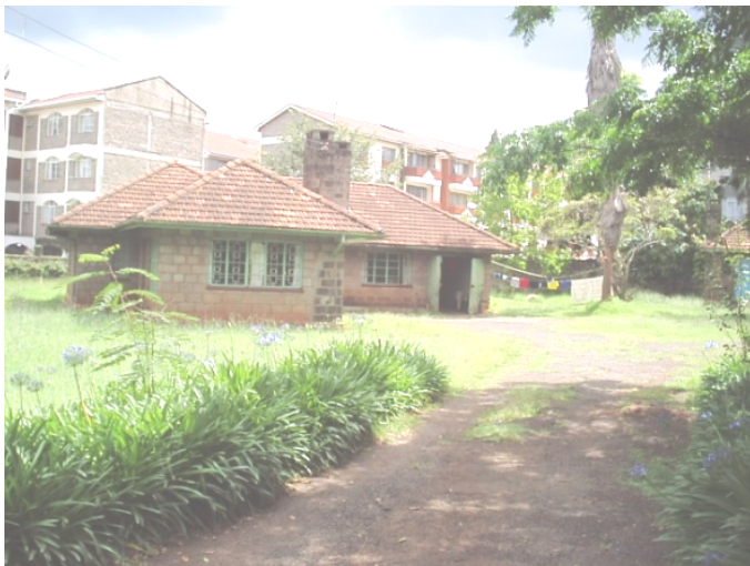
Plate 3.0-1 Pre-independence single storey houses along Manderu Road
