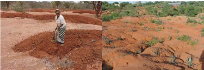
Plate 3 A woman digging soil and water conservation structures and sisal planted as a measure to rehabilitating Itivanzou gully in Kyuso.
