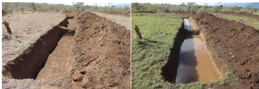
Plate 6 Established water retention ditches for rehabilitation of the Suswa gully in Narok.
