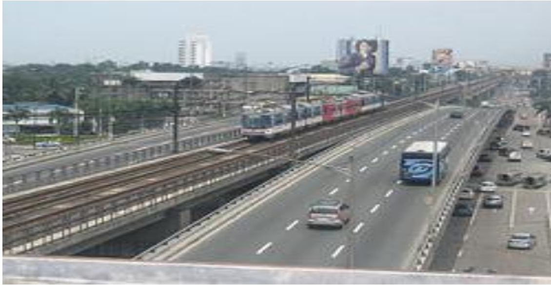
Figure 7: An MRT train in-between the EDSA-Quezon Avenue Flyover.
