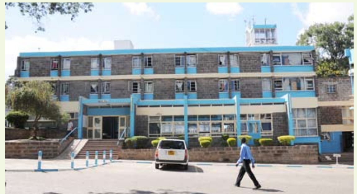
The Front elevation of Hall 9 also called Tom Mboya, named after the late Minister for National Planning and Economic Development.
