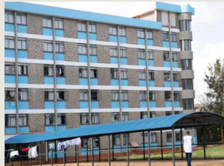
The completed Phase of Lower Kabete halls of residence.
