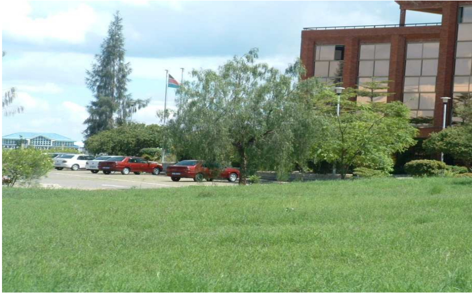
Plate 1: Administration building – Athi River EPZ Source – fieldwork August 2010
