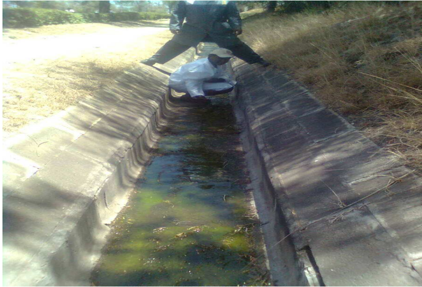
Plate 10 : The effects of delayed repairs- a drain with algae Source: Field work – 2010
