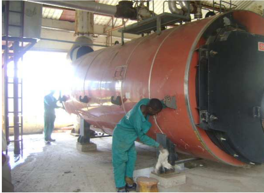
Plate 2 : Cleaning of boiler in progress Source: field work 2010
