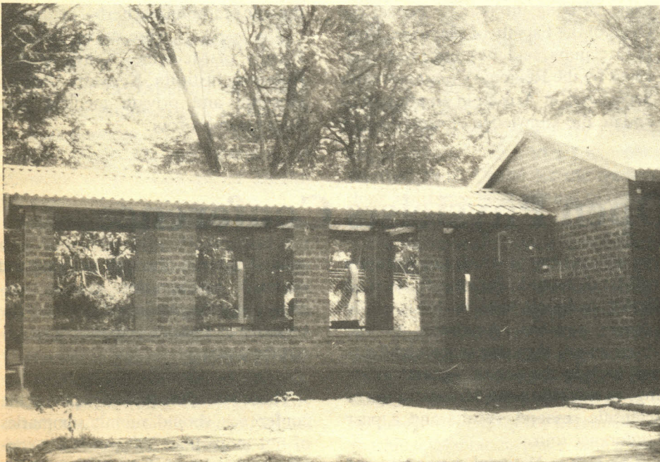
Low Cost housing unit developed by HRDU
