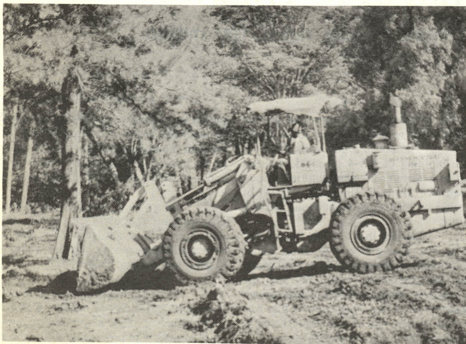
Preparing for 8-4-4: Constructing new laboratories at Upper Kabete campus
