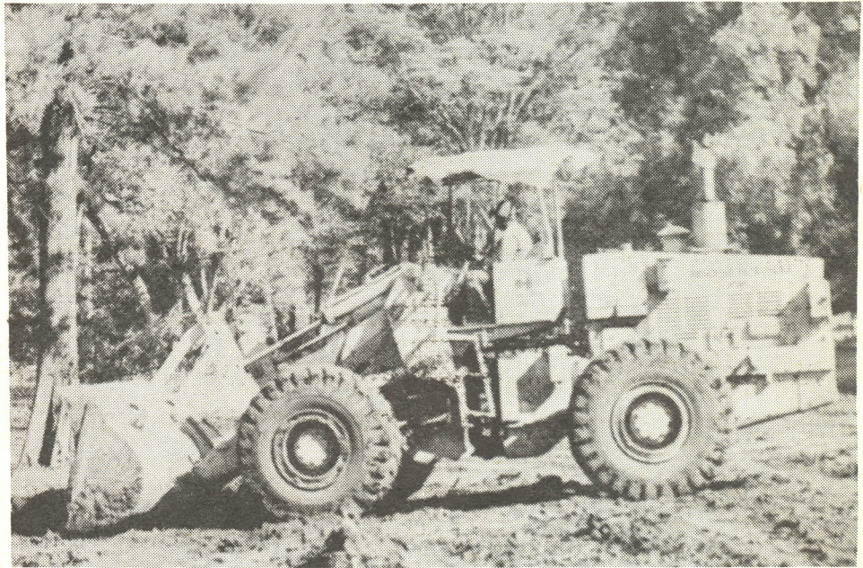
Building a giant: construction work on the new graduation venue.
