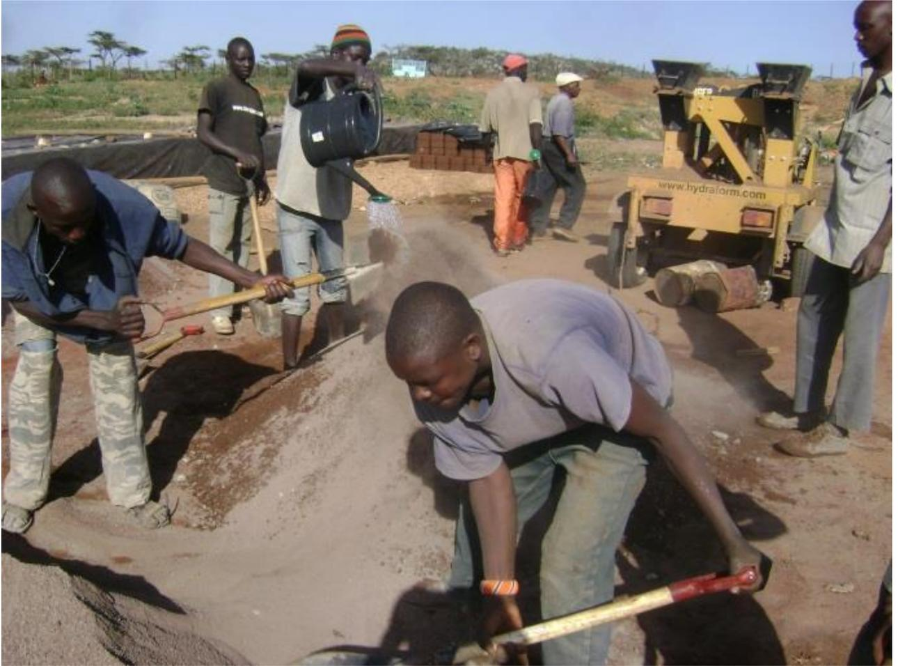
**Plate7: Material Preparation for ISSBs production**
