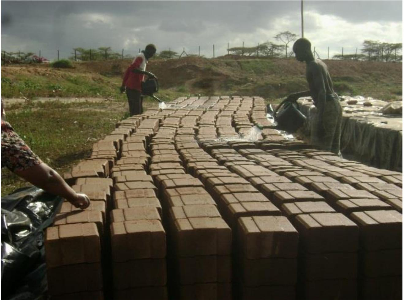
**Plate10: Curing of ISSBs at the yard**
