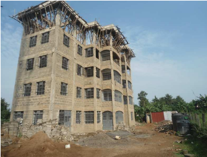
Figure 4.4: A two bedroom flat under construction in Amalemba estate.
