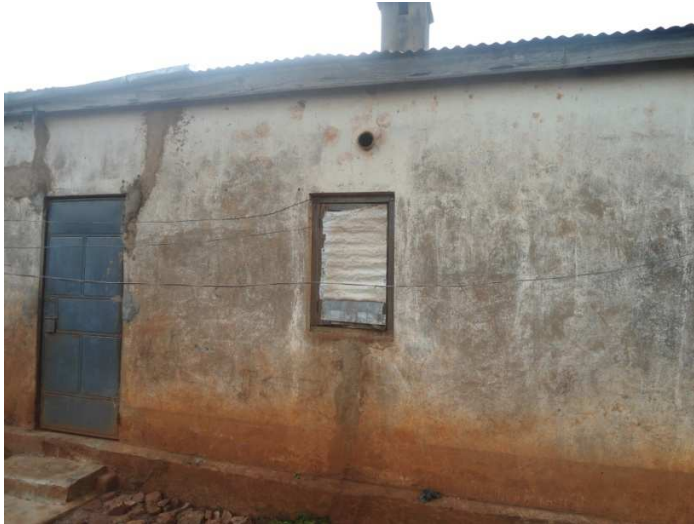
Figure 4.12: Low Grade Civil Servant House in Mudiri estate.
