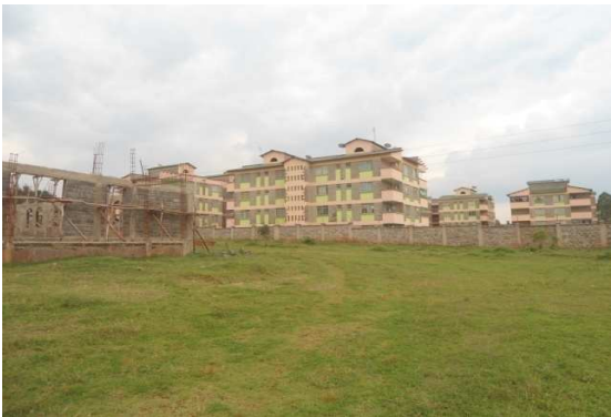
Figure 4.1: NHC flats at Amalemba estate.
