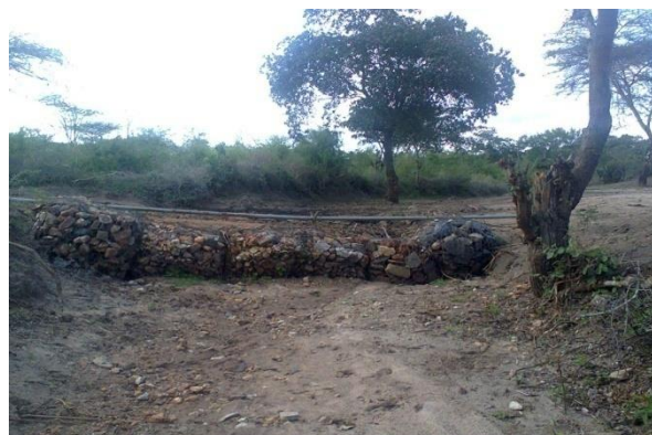
Plate 3.4: Gabions built for trapping sand Source: Field Survey, 2012
