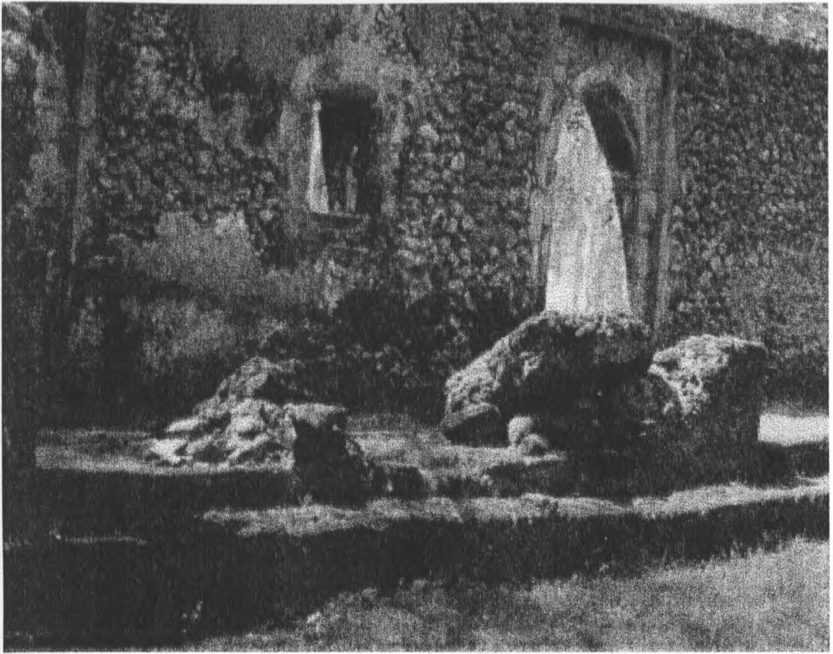
Plate 1: Rubbles of felled historic structure whose stones have been vandalized.
