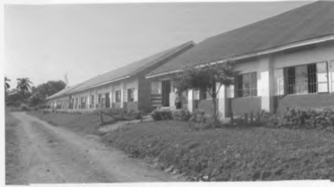
The researcher concludes at Ntare High School in Western Uganda
