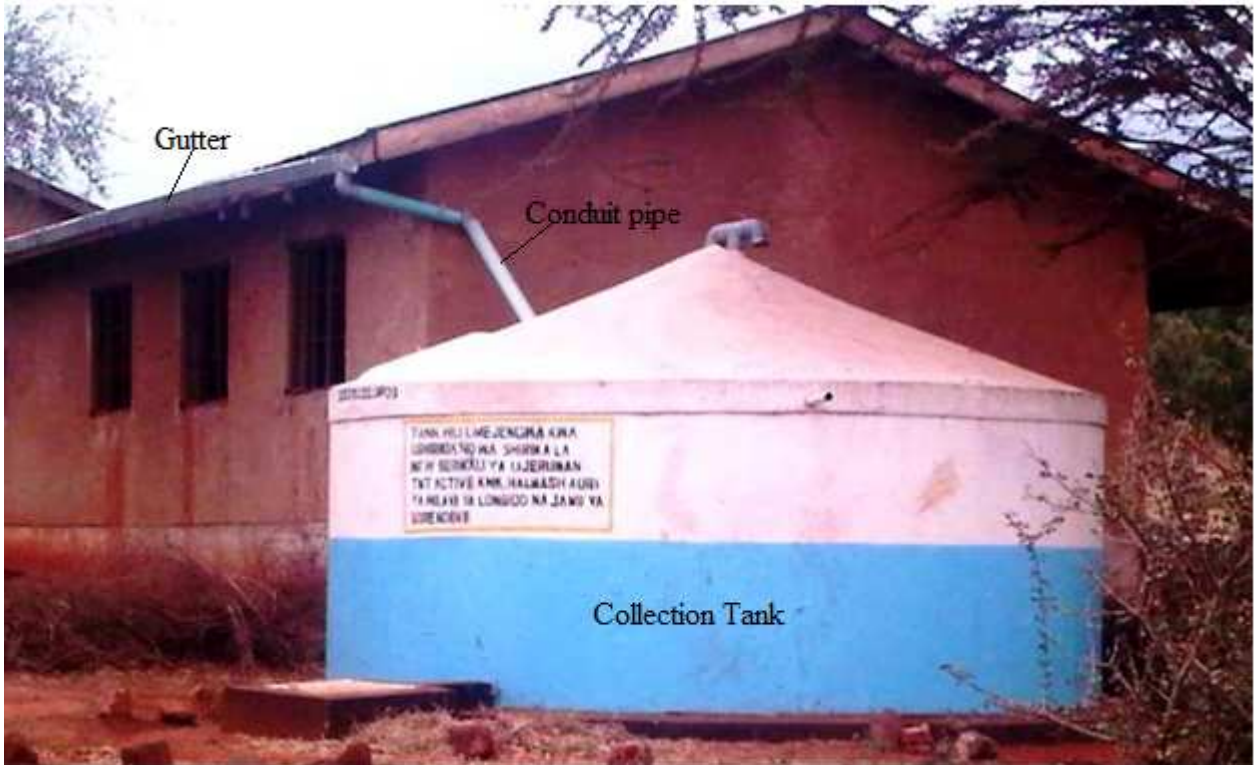
Figure 1: Picture showing rainwater harvesting system in public school, Longido District-Namanga (source: Field survey, July 2013)
