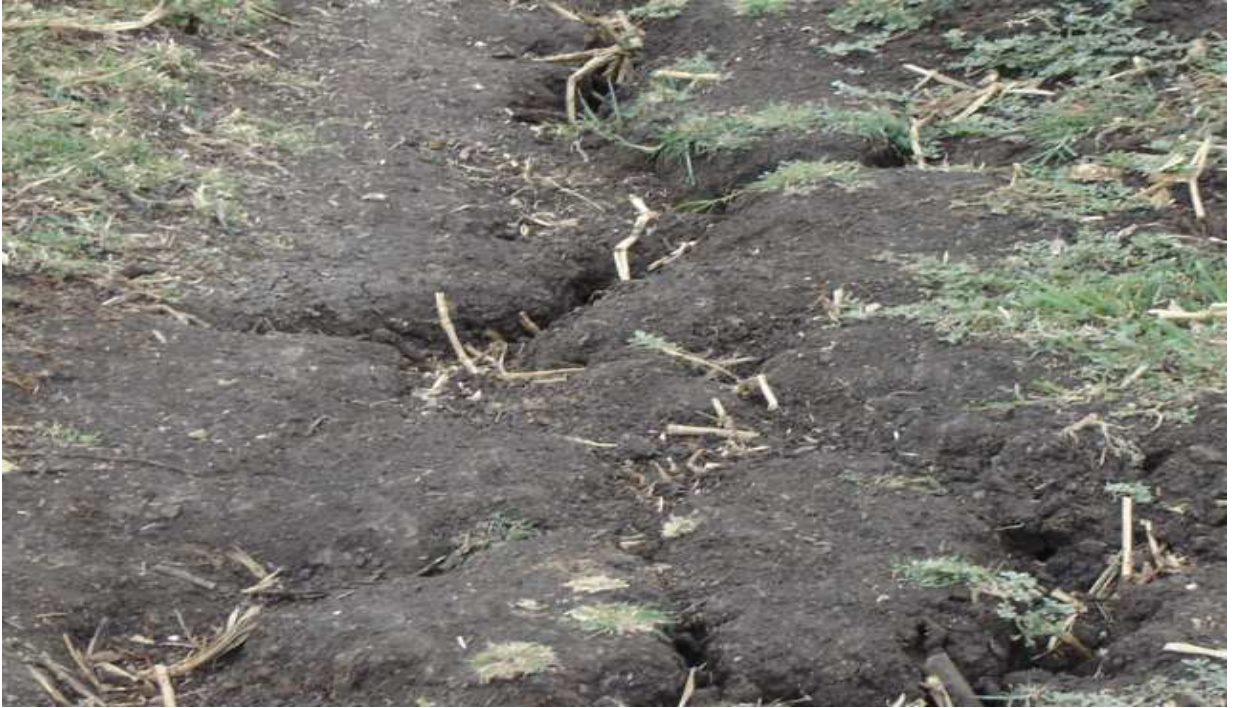
Photo 3 shows area with severe water erosion ( photo by kasenga )
