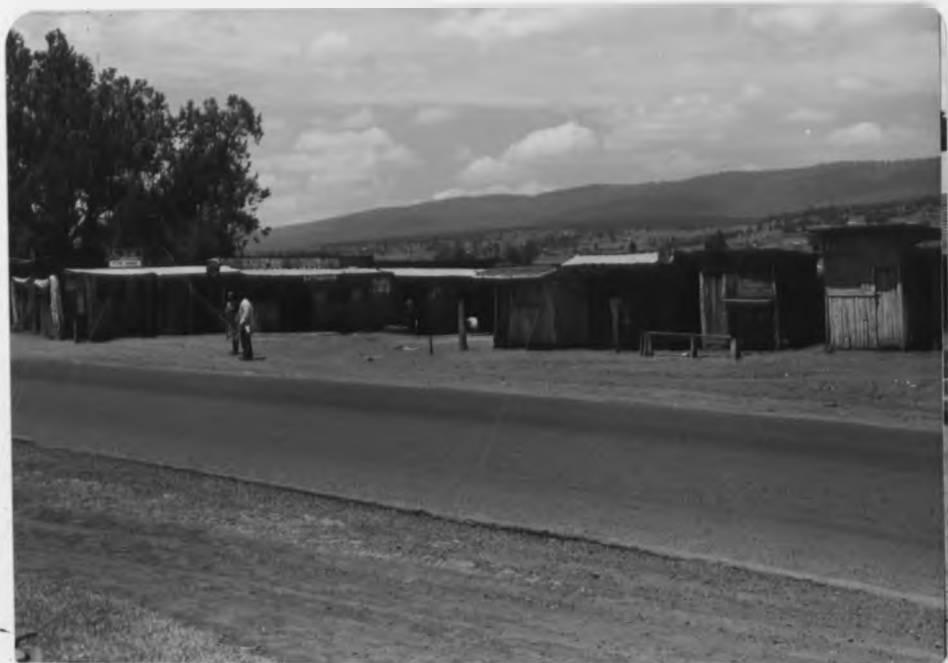
Plate 4: Kihingo non-designated centre in Mutukanio farm that has developed on a road reserve.
