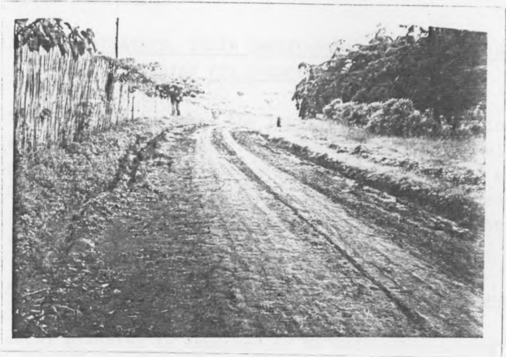
Plate 3. A section of the C19 Mbita-Homa Bay road. Notice the poor conditions of this section. Such sections make the road impassable in wet periods.
