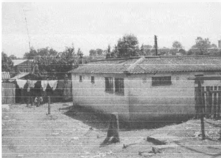
Fig. 3.6 Typical View of the Houses.
