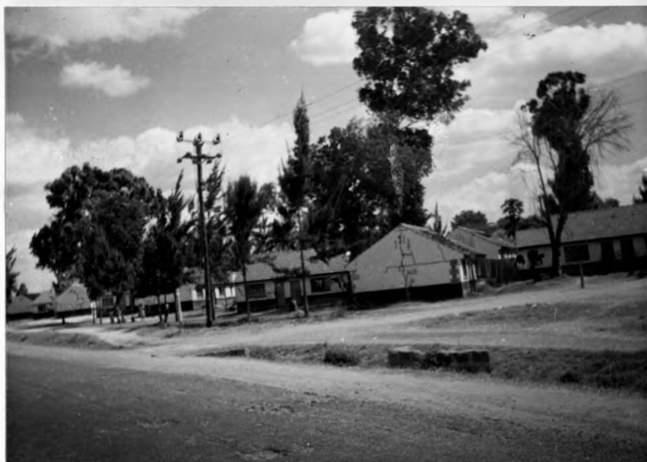
Makadara Council Housing. The notable repairs on the walls are a sign of the deterioration of housing in the estate.
