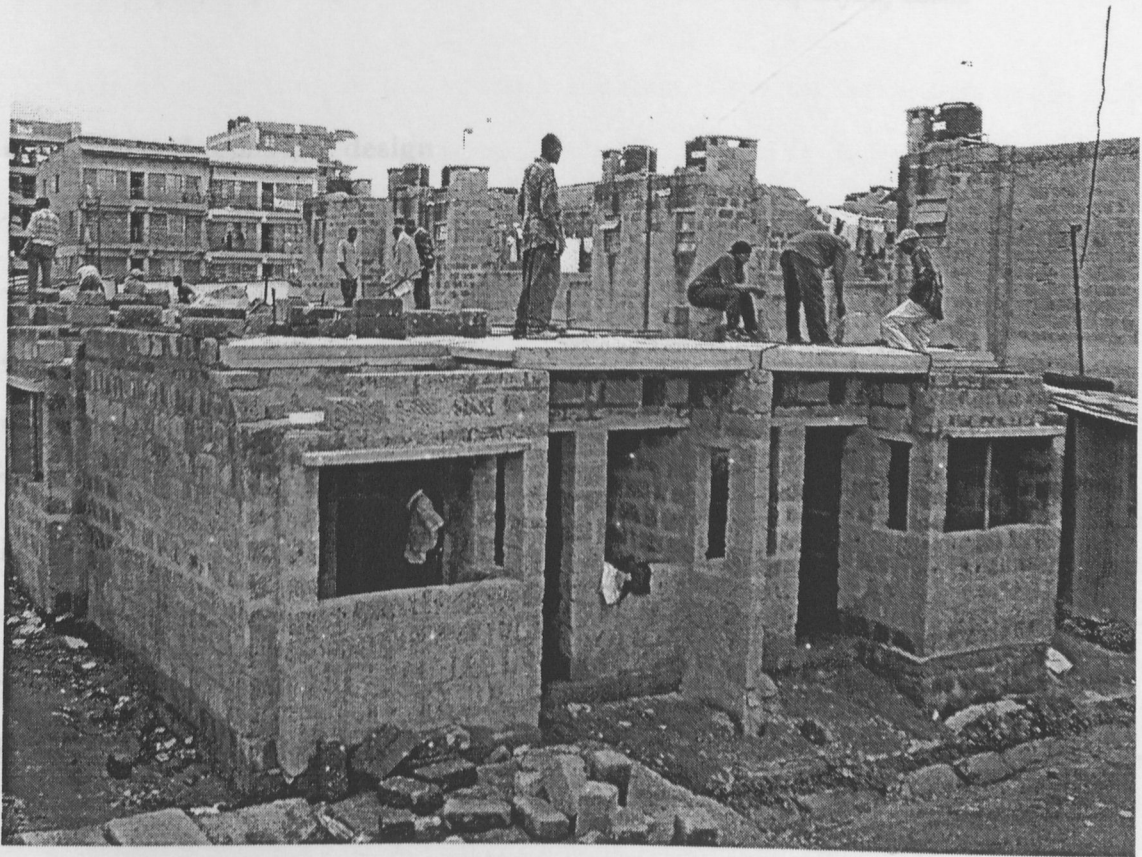
Fig.4.12 The upgraded houses under construction Picture by author
