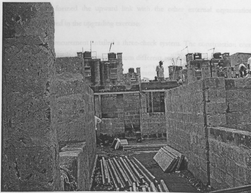
Fig.4.14 The construction site with the pre-cast concrete elements in the foreground
