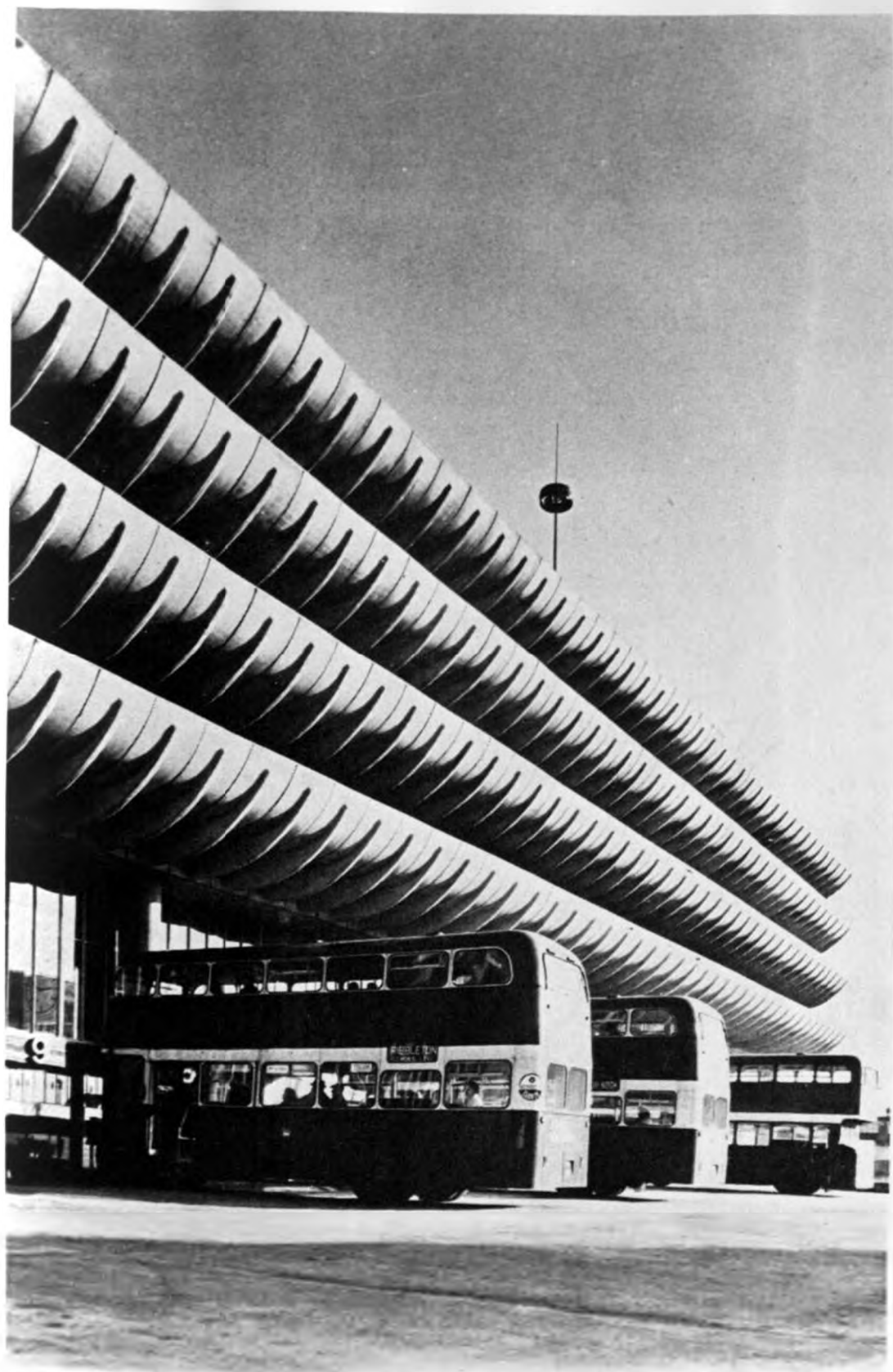
The cantilevered car deck project 2.74m to cover the passenger platform at concourse level.
