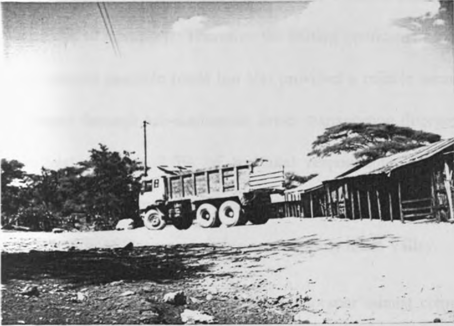
Plate 5.1: shows an All weather road constructed by KFC using fluorite bearing rocks. Notice that electrification and telephonization services have been extended to Kerio Valley.
