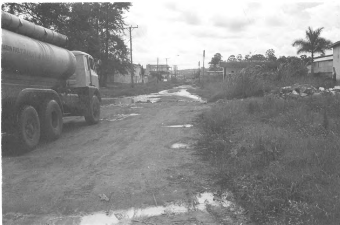
PLATE 3 Kibiira Road in Kampala Industrial Area. Impassable because of leakage of under-
