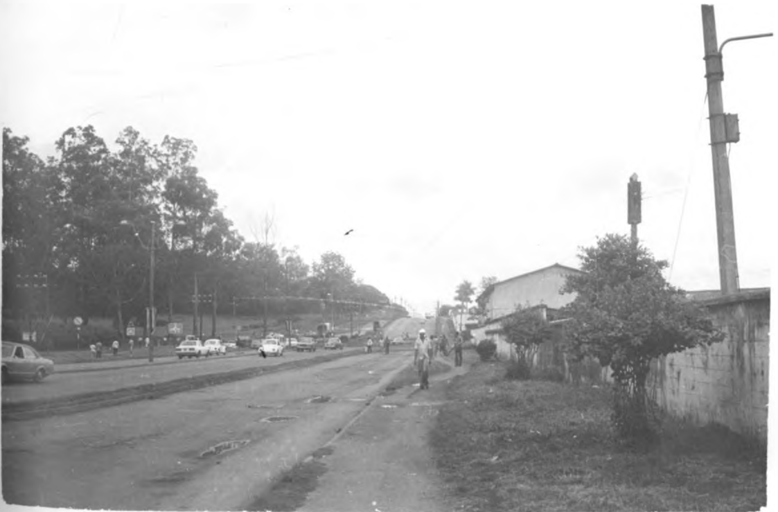
PLATE 10 Jinja Road. One of the roads serving Kampala Industrial Area.
