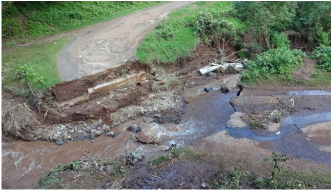
FIGURE 6 A bridge destroyed by the mudslide along Thingitungi stream.
