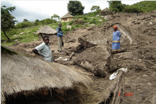
FIGURE 9 House destroyed by huge rock boulders down a slope due to a landslide.
