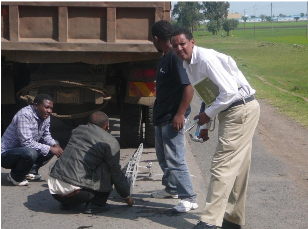
Figure 3-6 Deflection measurement using Benkelman Beam on Progress
