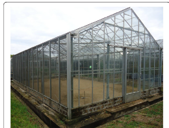
Figure 1 The semi-field system at icipe-Thomas Odhiambo Campus, Mbita, Kenya.
