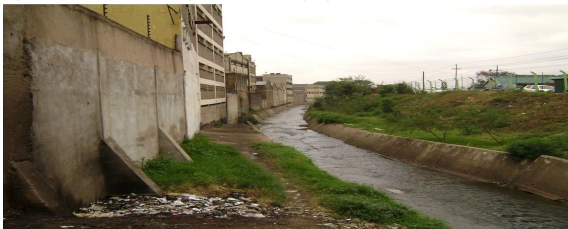
Figure 7.1: Industrial Buildings on Canalized Ngong River.
