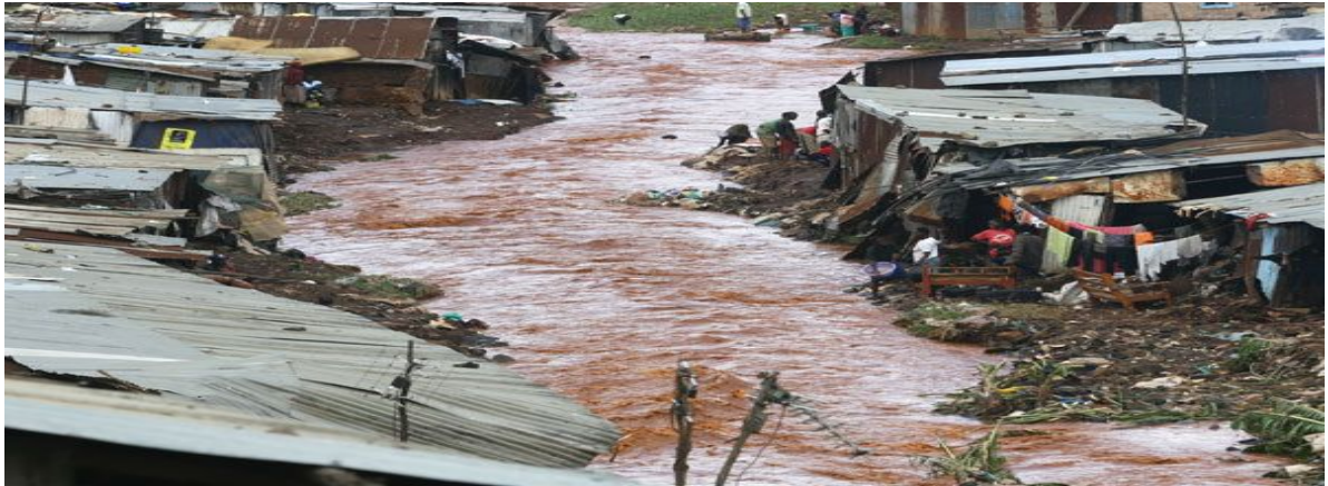
Figure 7.5: Structures Constructed at the Edge of Mathare River in Mathare 4B
