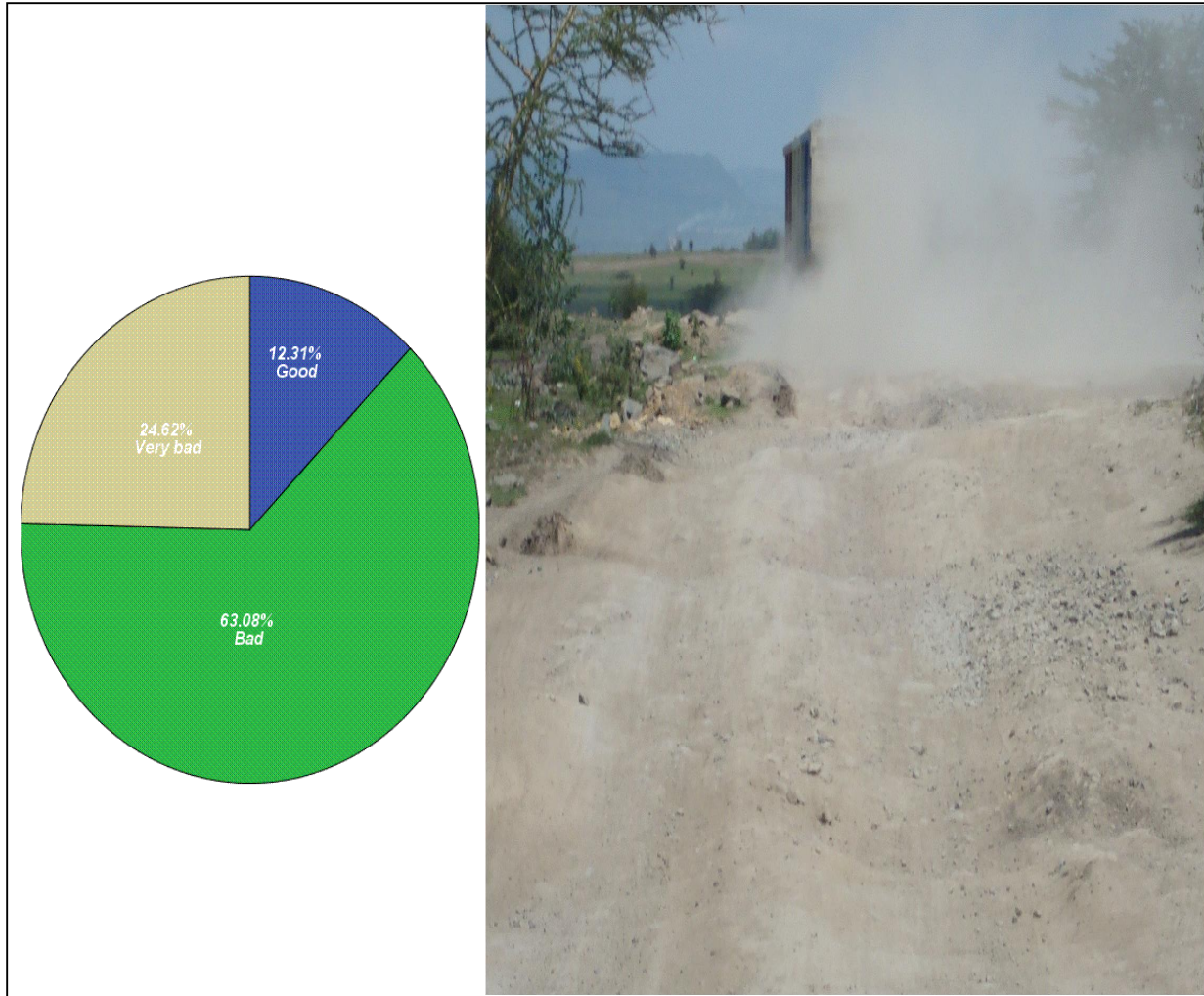
Figure 13: Condition of roads: Source: Field survey, 2014
