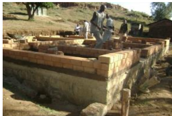
Plate 6: ISSBs construction process
