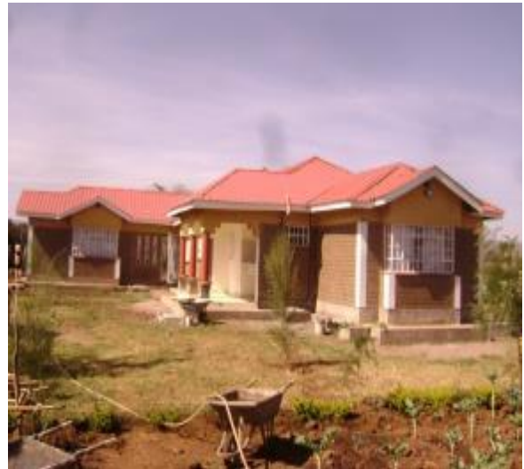
Plate 8: ISSBs constructed residential house
