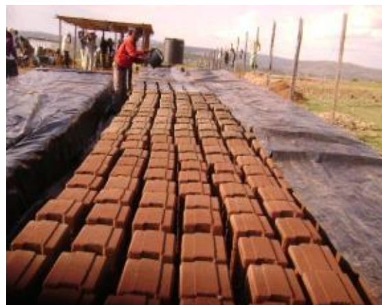
Plate 6: ISSBs construction process
