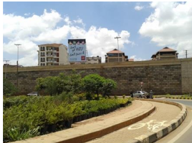
Plate 27: Limuru Road and Forest Road Interchange
