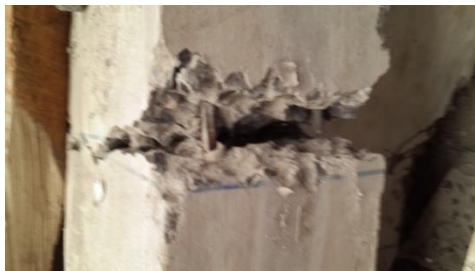
Figure 7: Snap steel tensile reinforcement
