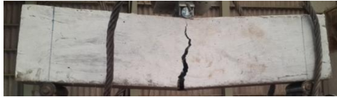
6.1: Failure pattern of L.B. 805
