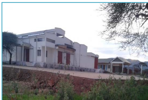
KMC Slaughter House under construction at Isiolo County
