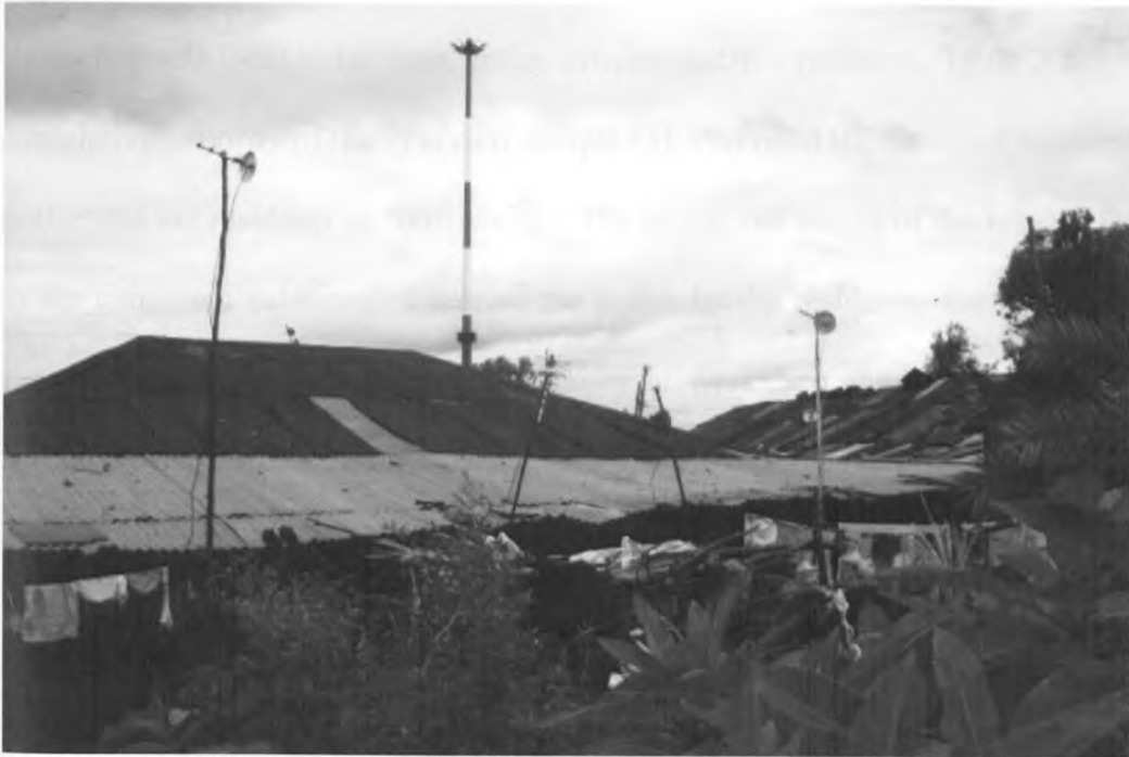
Figure 10: High mast flood lighting to complement electric power lines
