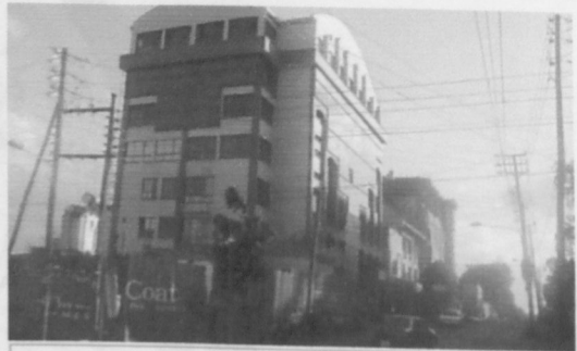
The office building has three extra floors (October 2011)
