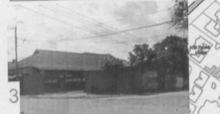
3 CHANGE OF USE: Residential houses have been converted to hostels
