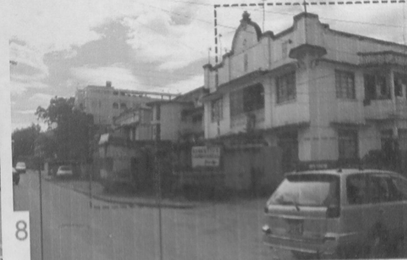
8 CHANGE OF USE: conversion of residential to hostels ● Informal Kiosks encroaching into the main roads
