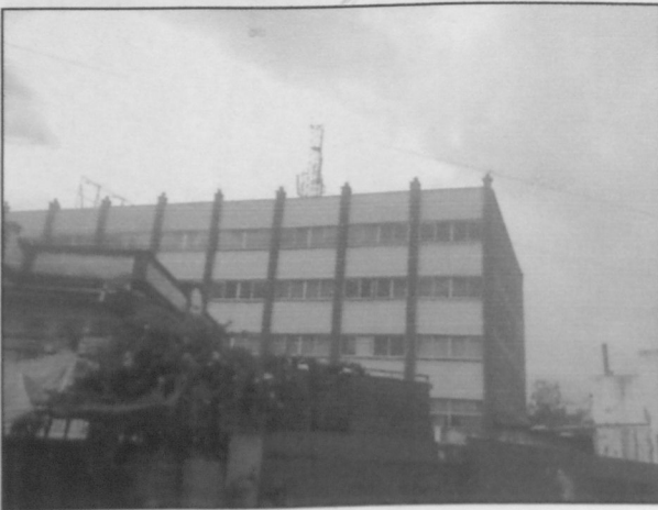
Fig. 5.7 Original built form. Source: Author, 2010.
