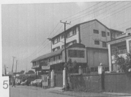
5 TOTAL CONVERSION: Formerly a residential house remodelled to accommodate a restaurant and a pub in the first two levels and hotel rooms on the upper levels.
