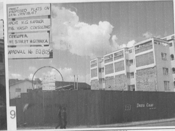
9 DEMOLITIONS AND RECONSTRUCTION: Demolishing residential dwellings for High-Rise flats
