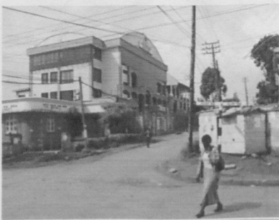
The two plots before the transformations (June 2010)
