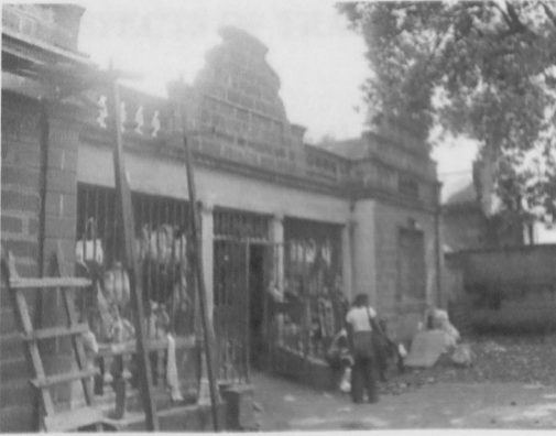
Fig. 5.30: Front facade of the 1929 Indian type dwelling house undergoing gradual transformations both at house level and plot level, extension at the rear. Source: author
