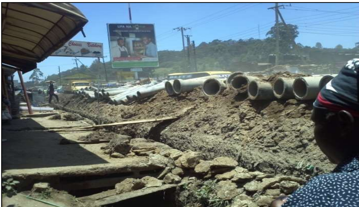
Plate 5.17: Drainage system under construction in Mutuini.
