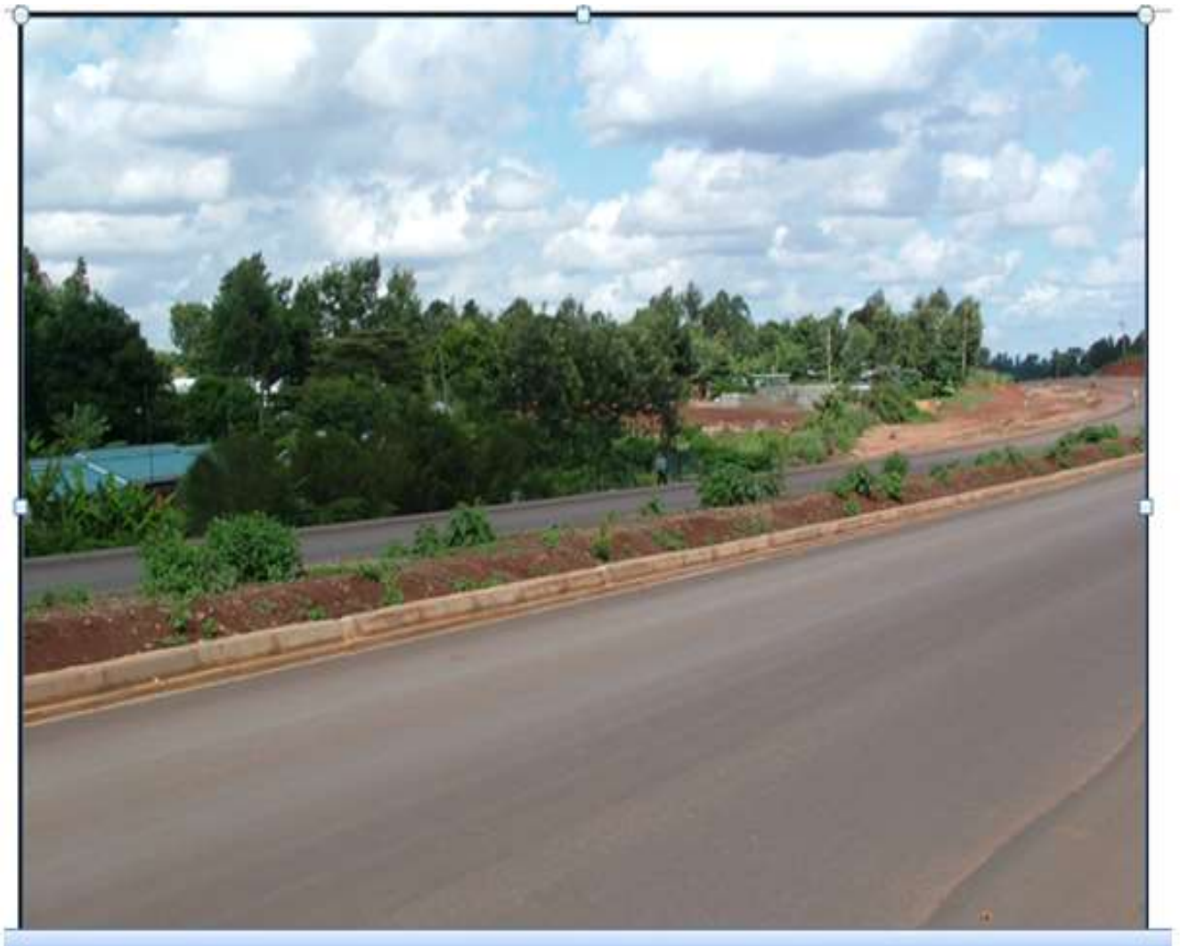
Plate 4.5: Southern-Bypass construction through Mutuini.
