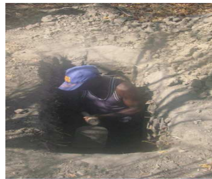
Plate 3.5 Excavation of open pit
