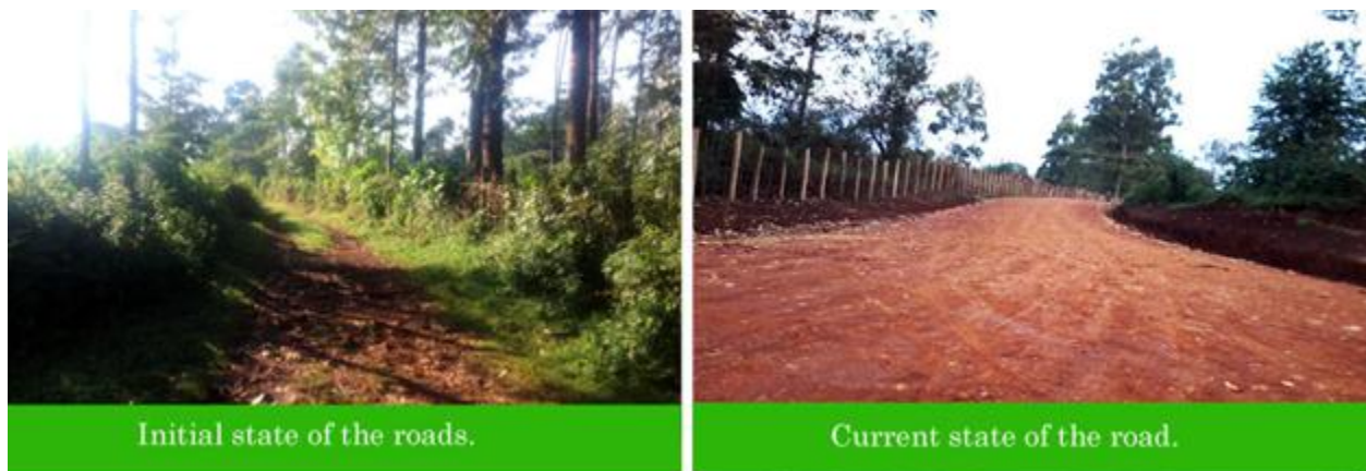
Figure 2.3: Initial state of the access road and the current state
