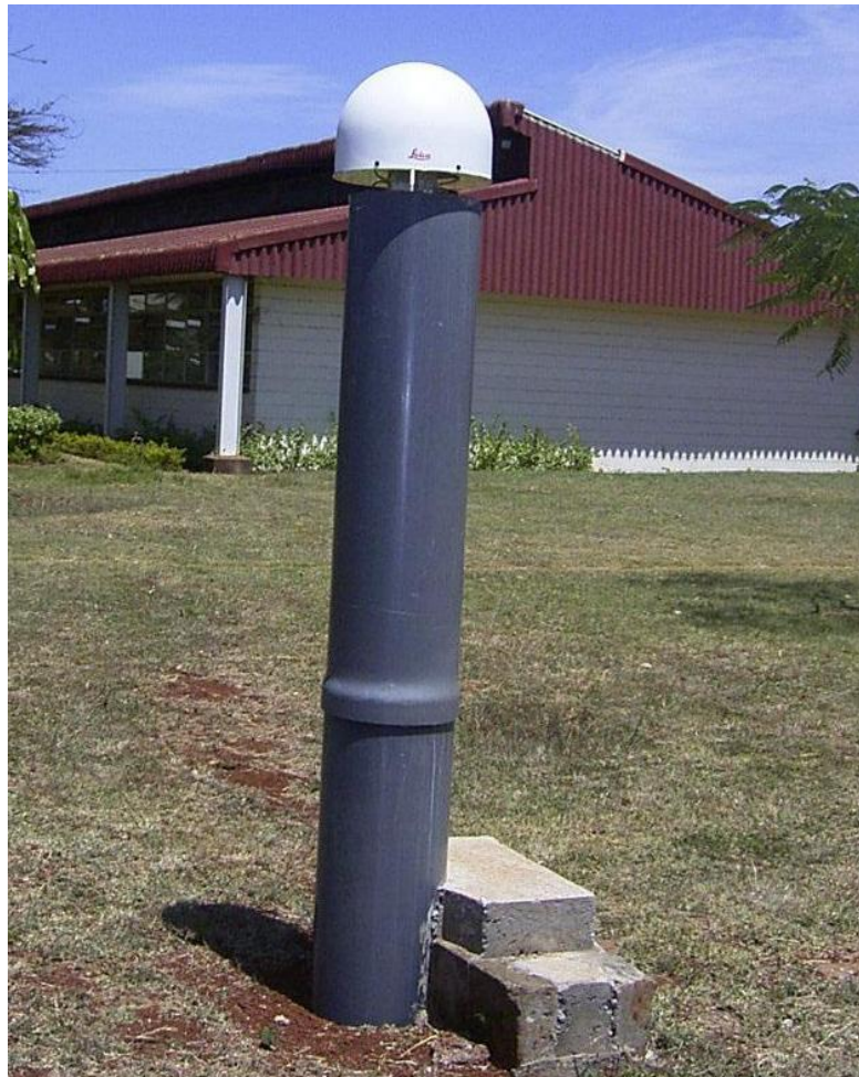
Figure 4-1: GPS Antenna at RCMRD, the GPS Receiver is housed in RCMRD Office in the background.
