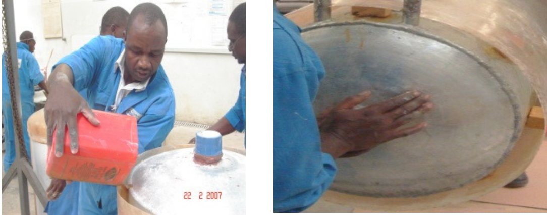
Figure 1.2: Galvanized Tank inside GRP Barrel Being Insulated ( Courtesy: D&S, 2014).
