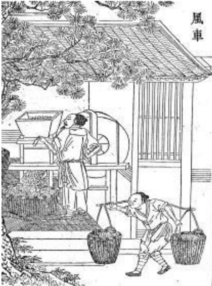
Air Separation, 1,500 AC China
