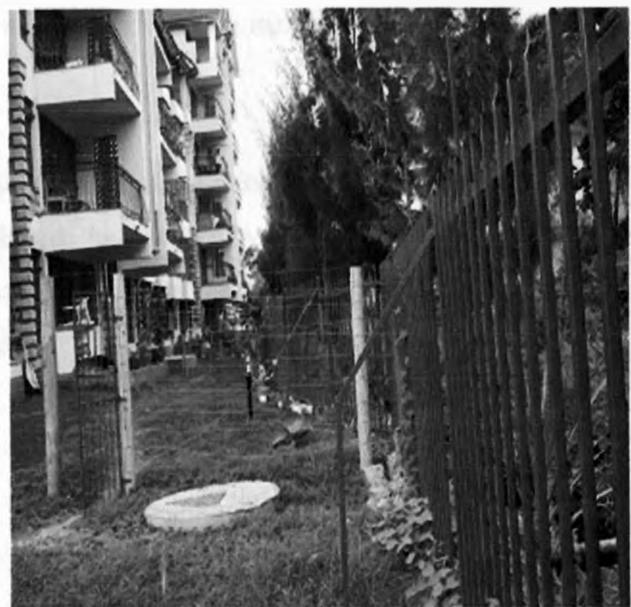
Apartment encroaching on Riparian reserve
