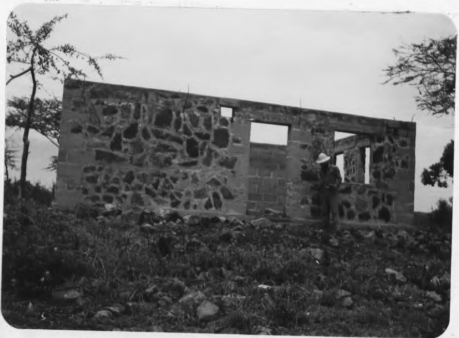
Plate 2: Wall construction using locally available natural stone.
