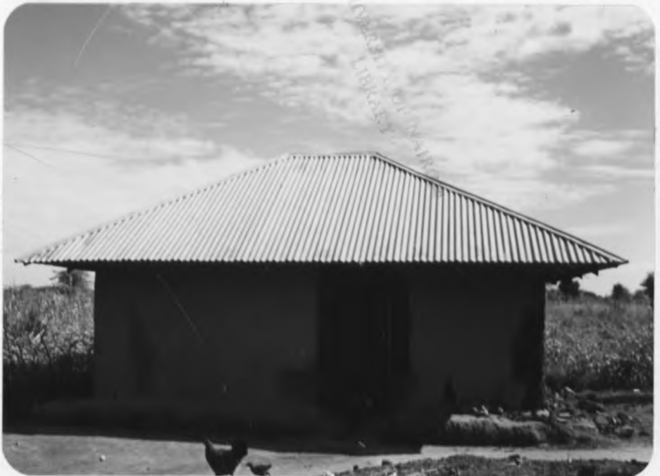
Plate 8: This house shows a combination of "modern" building materials (corrugated iron sheets) and traditional materials (Clay and cow-dung) for walling.
