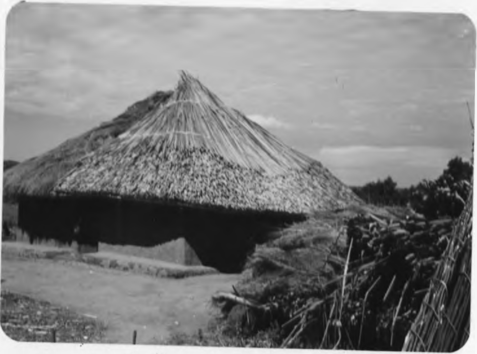
Plate 3: Reeds replacing grass as roofing material. The re-roofing is still half-way through.
