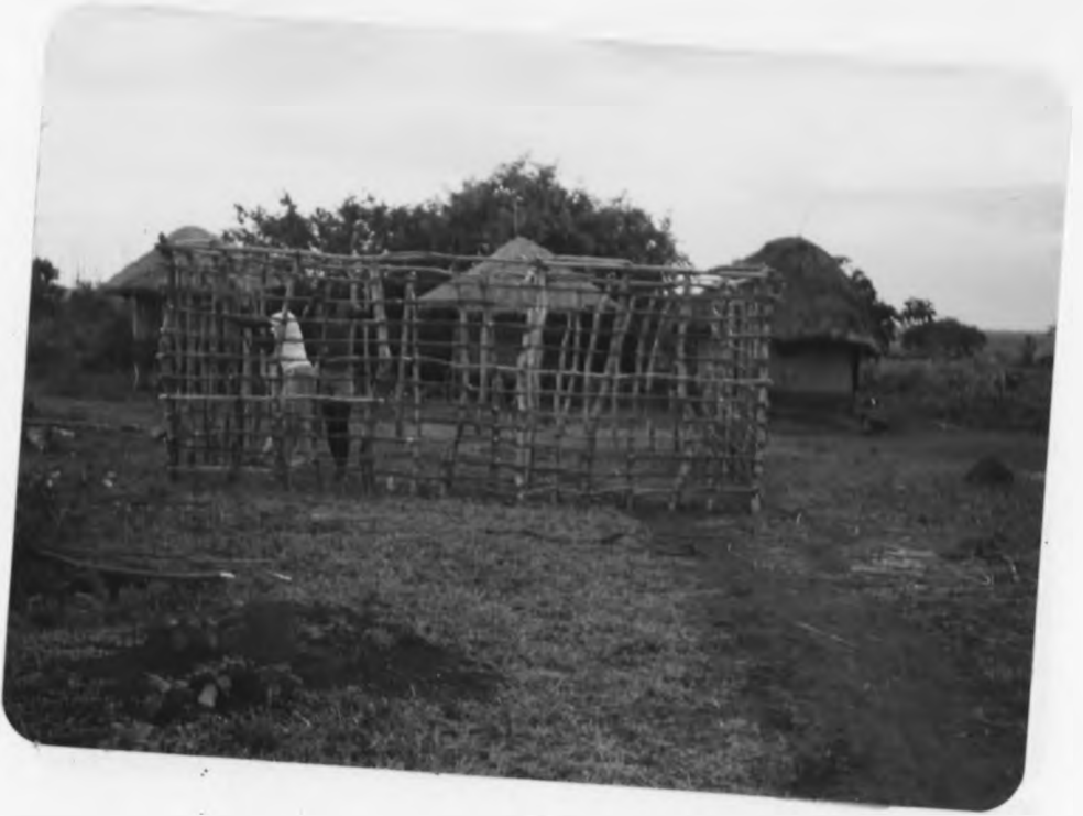
Plate 1: Wall construction using traditional methods and skills.
