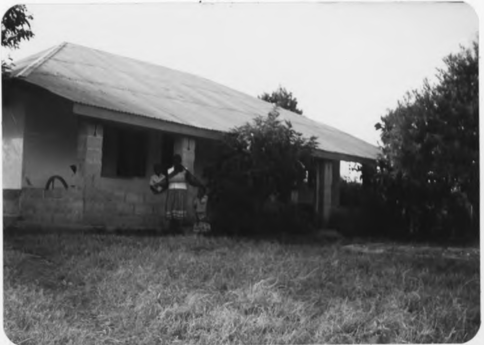
Plate 10: An example of adequate house constructed using concrete blocks in some rural areas of Siaya District.
