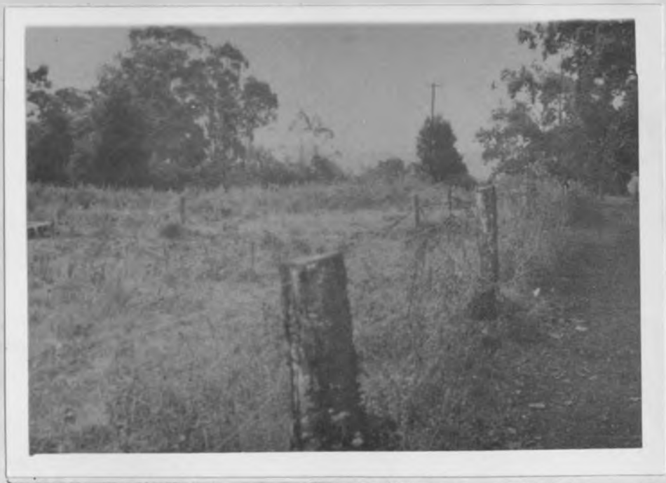
Fig. 3. Loose wire fence seen supported with thorny bushes after clearing.
