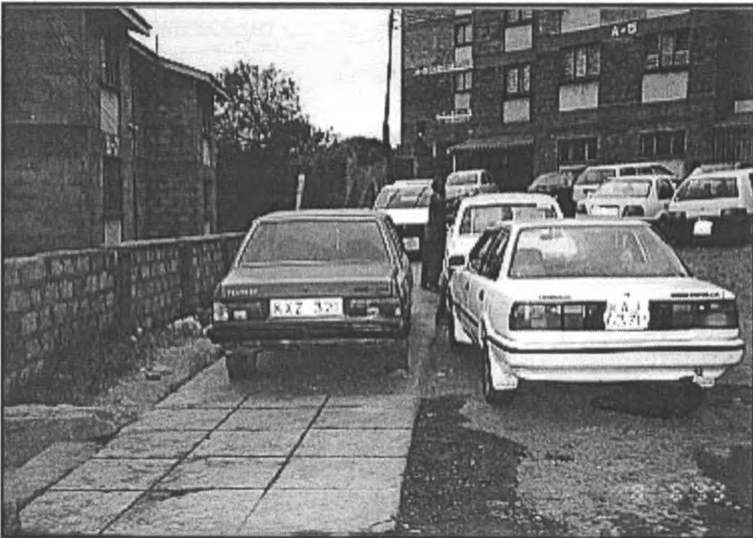
PLATE 5: Kerb parking that hinders pedestrians accessibility
