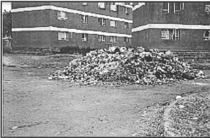
PLATE 9: Garbage Disposal on the Circulation space – Parking space
