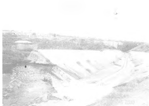
Meshed gabion recently constructed to control storm water carrying waste inflow and a concreted out spill that is in a good working condition.
