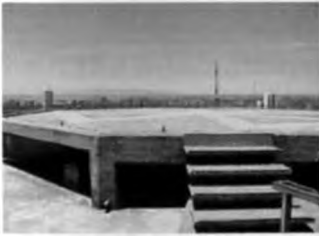
Fig 2.5: Helipad at K.I.C.C
