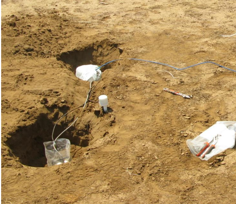
Figure 4.3: Field deployment of equipment
