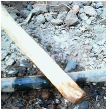
Fig. 4.4(g) Knocking of clogged emitter using a short peg
