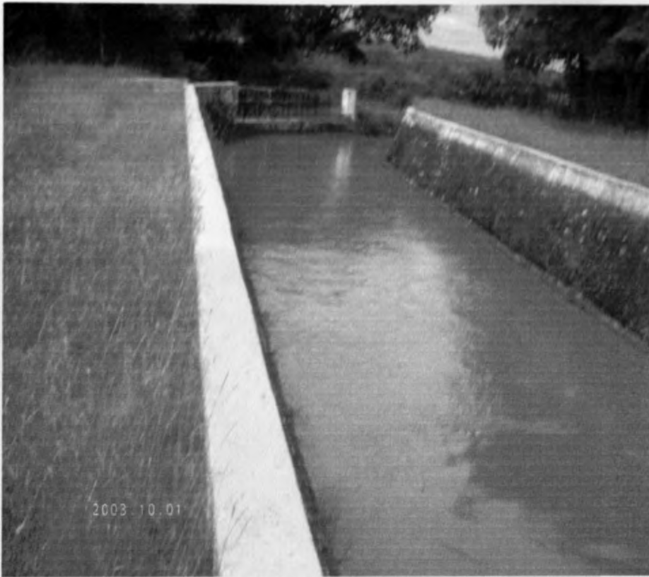
Figure 1.2 The Yatta Canal Immediately after the intake point.
